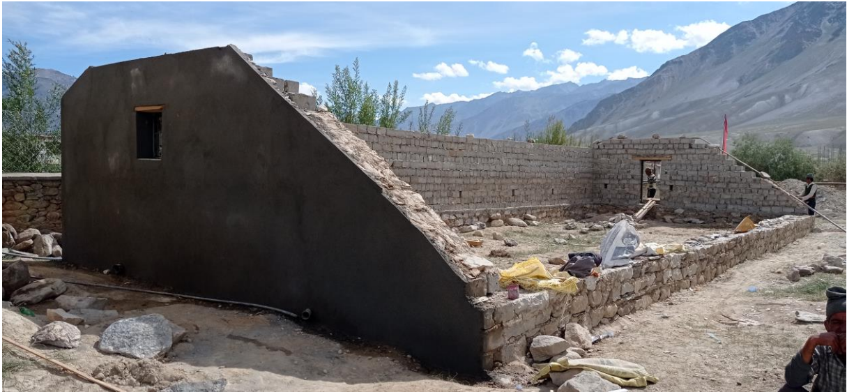
Figure 22 serre -work in progress
